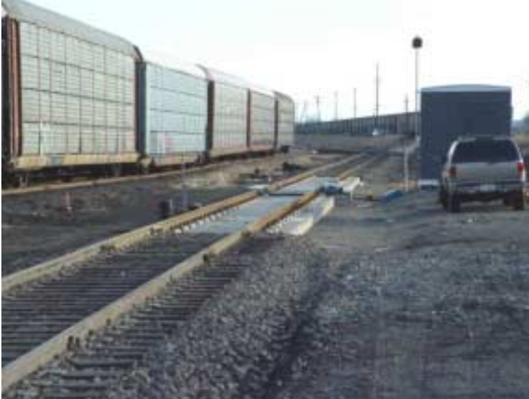
North Shore Rail Group weigh-in-motion scale, Williamsport, PA. 1/6/2004. Note auto racks, a rarity on shortlines.
