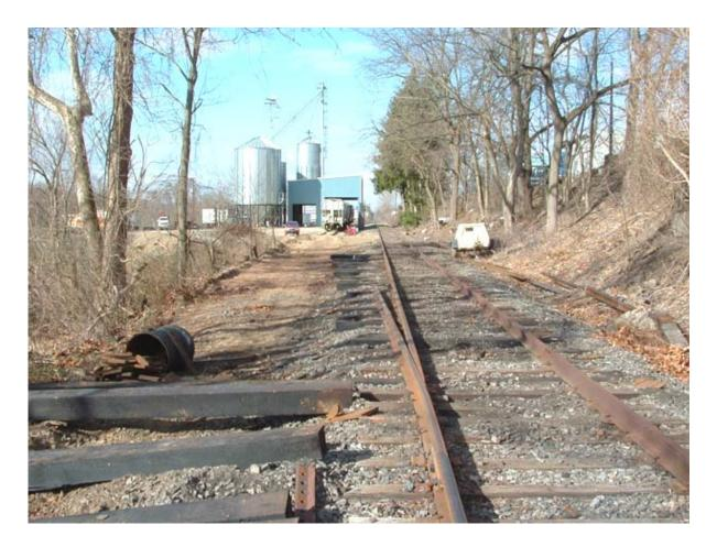
New switch and siding extension at Brandt Flour Mills transload facility in Lime Ridge, PA on NSHR. MP 181.7.
