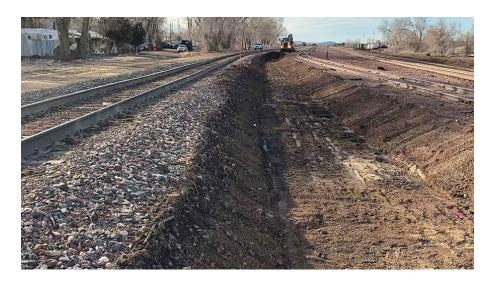
This track bed excavation is for a siding extension project on the Phoenix line at Ash Fork, Arizona, just south of the Williams junction on the ex-Santa Fe transcon. Genesee & Wyoming's Arizona & California short line, winner of the BNSF Short line of the Year award, joins the Phoenix line at Wickenburg.
